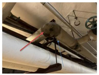
Photo 13 Thermal System Insulation (ACM)
