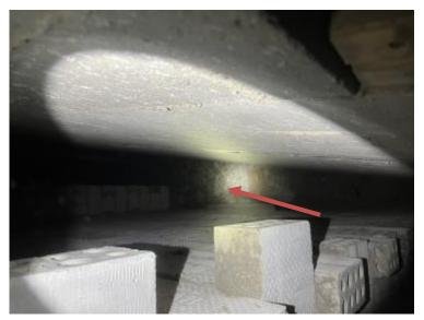
Photo 29 Acoustical Plaster Debris Below Catwalk (Assumed ACM)
