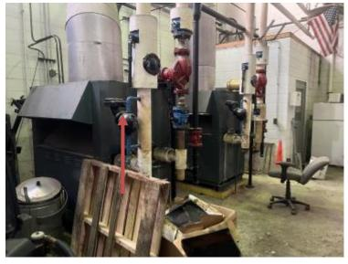
Photo 16 Interior Boiler Components (Assumed ACM)
