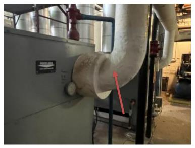
Photo 17 Boiler Breaching (ACM)
