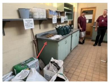
Photo 25 Asbestos Cement Tabletop (ACM)
