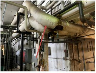
Photo 14 Thermal System Insulation (ACM)
