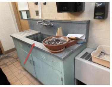
Photo 26 Asbestos Cement Tabletops (ACM)
