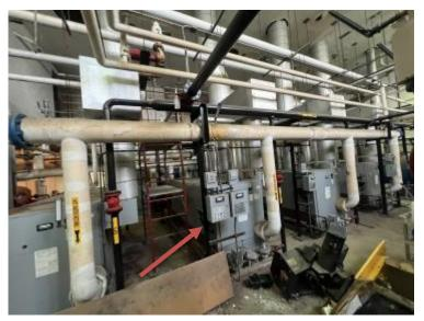
Photo 21 Interior Boiler Components (Assumed ACM)
