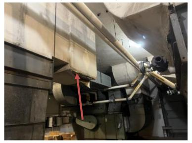
Photo 11 Duct Pin Mastic (Assumed ACM)
