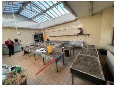
Photo 24 Asbestos Cement Garden Beds (ACM)
