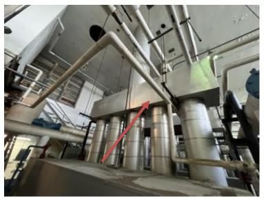
Photo 22 Boiler Breaching (ACM)
