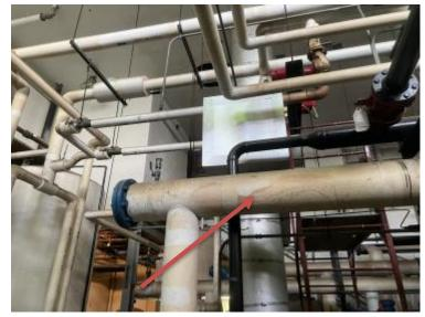
Photo 20 Boiler Breaching (ACM)
